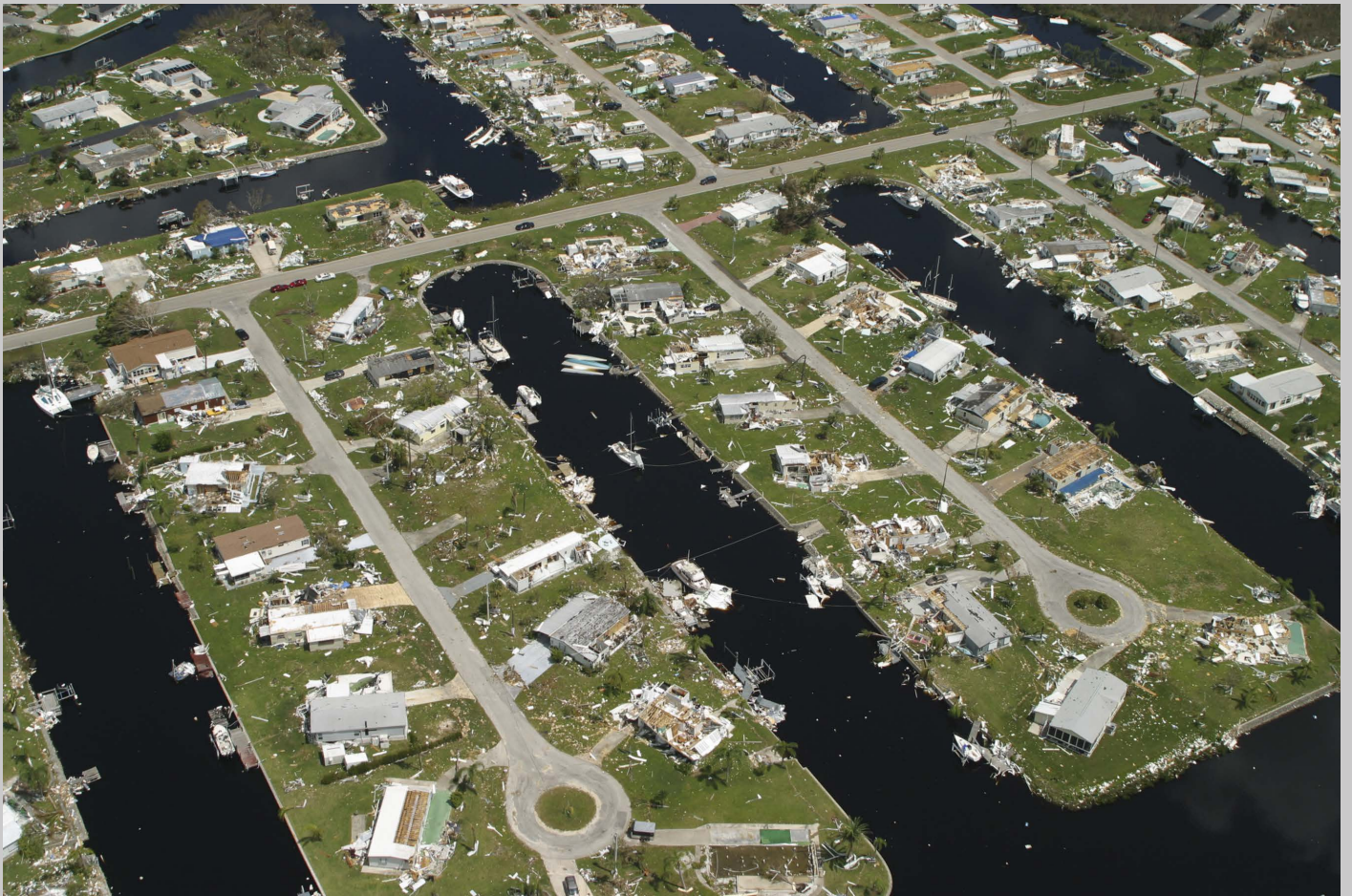
Aerial view of damage from Hurricane Charley suffered by a mobile home park in Punta Gorda, Florida, 2004.
